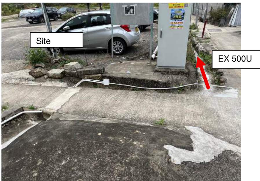
Photo 3 – Site Condition (Feb 2025)
