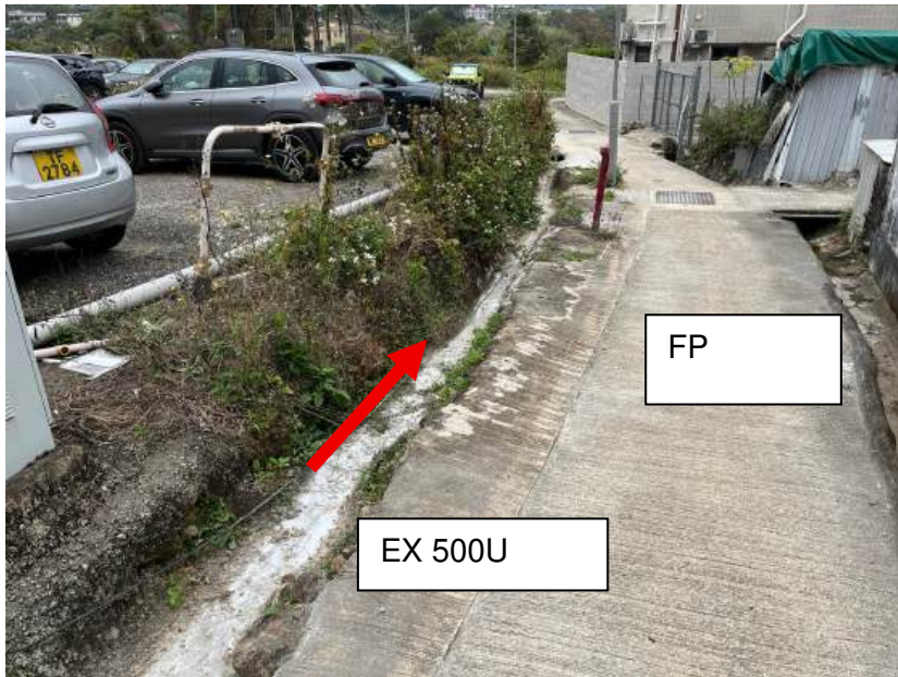
Photo 4 – Site Condition (Feb 2025)
