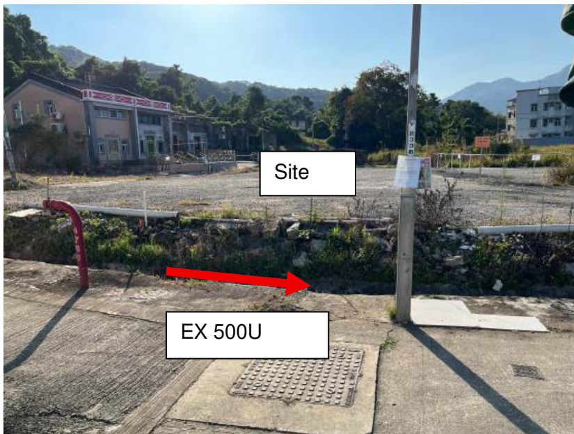
Photo 2 – Site Condition (Dec 2025)
