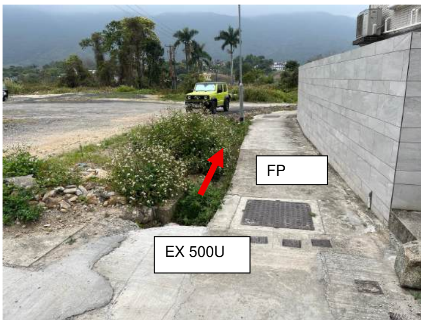
Photo 5 – Site Condition (Feb 2025)
